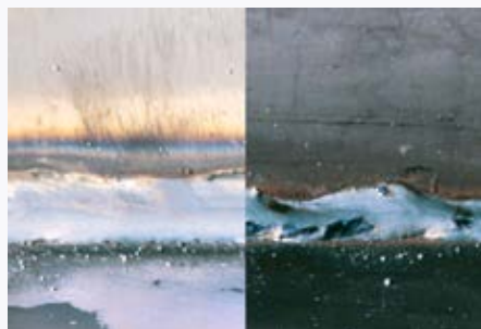
Surfaces descaled prior to welding result in clean welding seams (see image at left)
