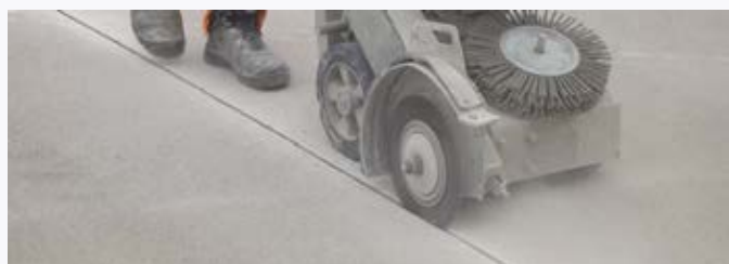
Joint brush used in road construction
